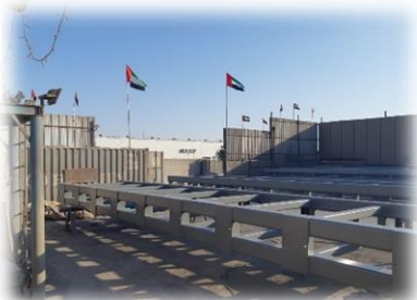
Fujairah Business Center – Heavy Structural Steel Project
