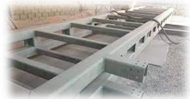
Heavy Structure – Fujairah Business Center Project
