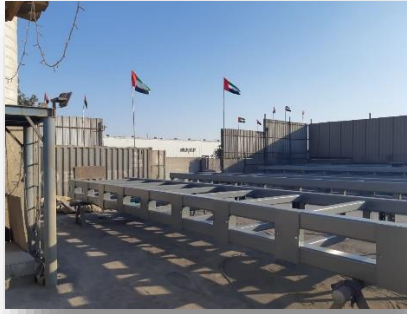
Fujairah Business Center – Heavy Structural Steel Project
