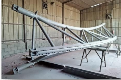
Heavy Steel Structure – School Project In Al Ain
