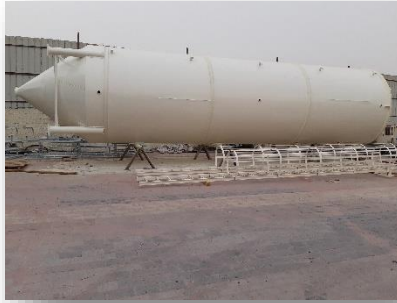
Silo – Cement Factory
