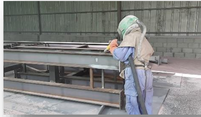
Heavy Structural Oil & Gas Project
